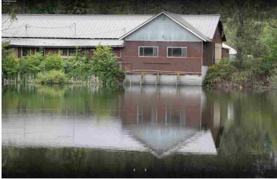
Figure 43. Derelict Warehouse & Pond
